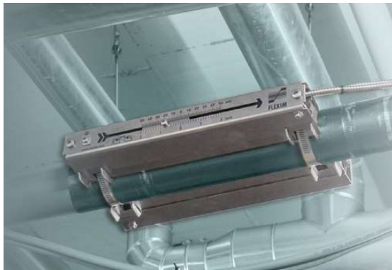
Ultrasonic compressed air flow meter
