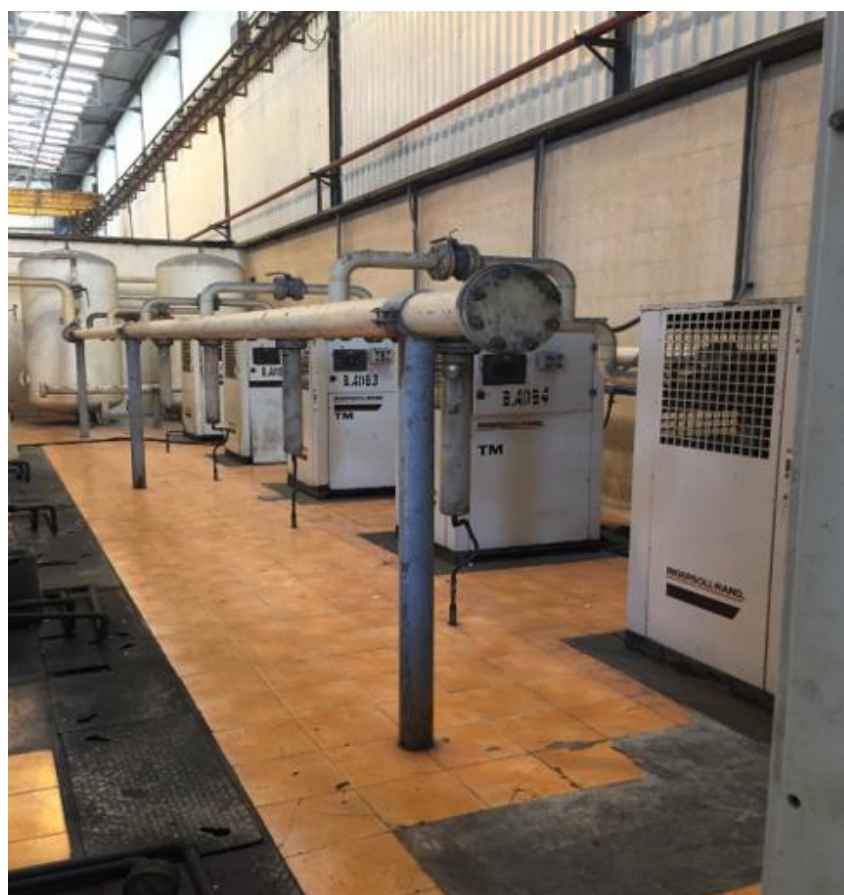
Figure 14-58: Air dryers
