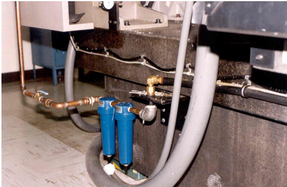
Figure 6-5: Examples of Point of Use Piping
