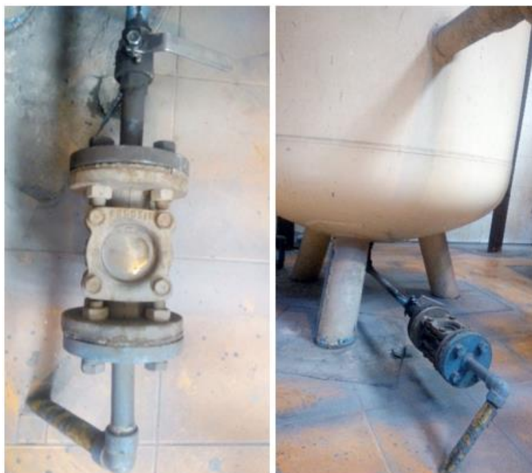
Figure 14-61: Manual drain valve for wet tanks
