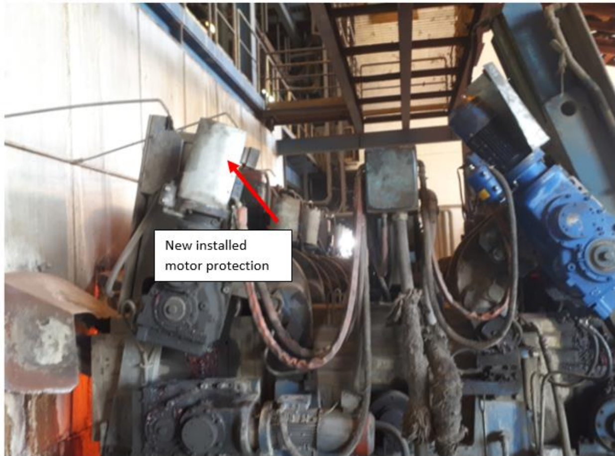
Figure 14-19: Withdrawal motors after new covers were installed (after remedy action)
