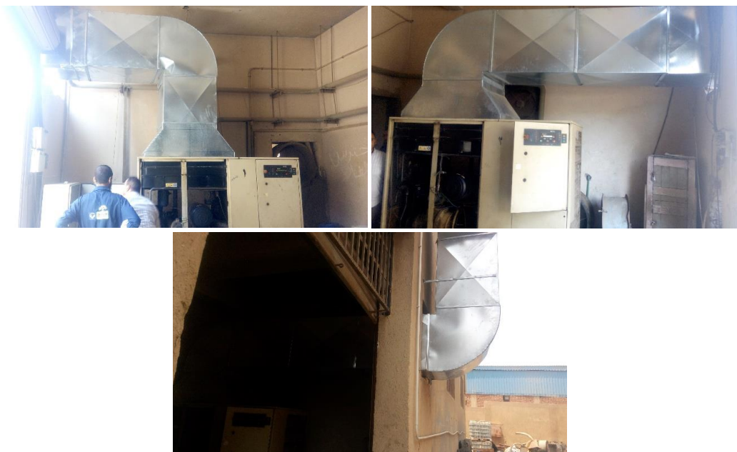
Figure 14-56: Newly installed ductwork to improve operating conditions in compressor room
