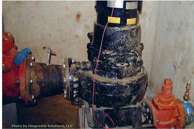
Fig. 12.16. Taps for Measuring Suction and Discharge Pressure
