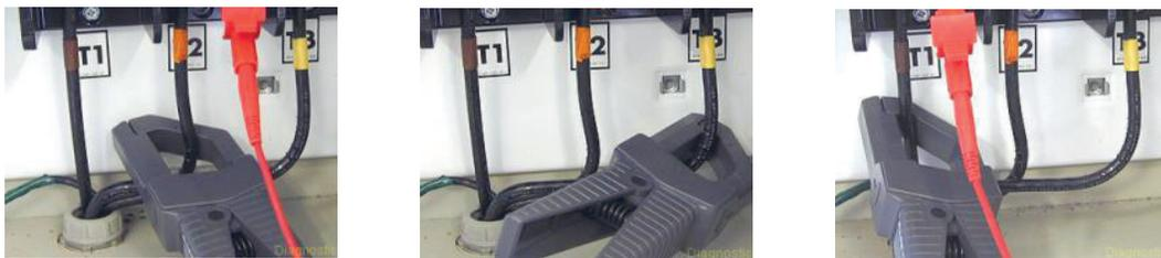
Fig. 12.28. Monitoring all Three Phases
