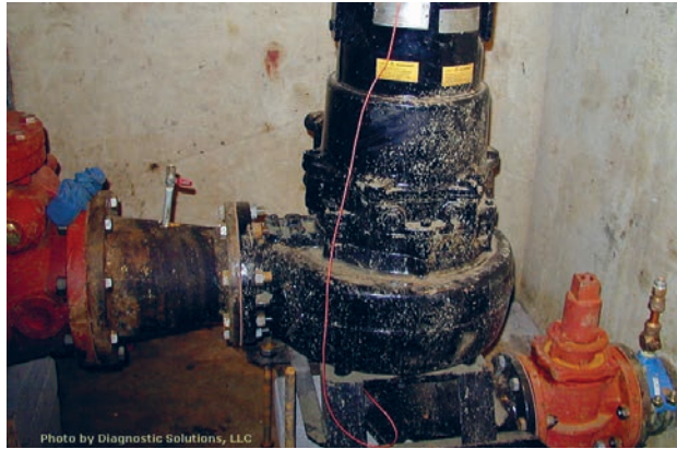
Fig. 12.16. Taps for Measuring Suction and Discharge Pressure
